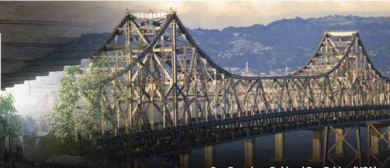
San Francisco Oakland Bay Bridge (USA) Structural Health Monitoring provided by MISTRAS
