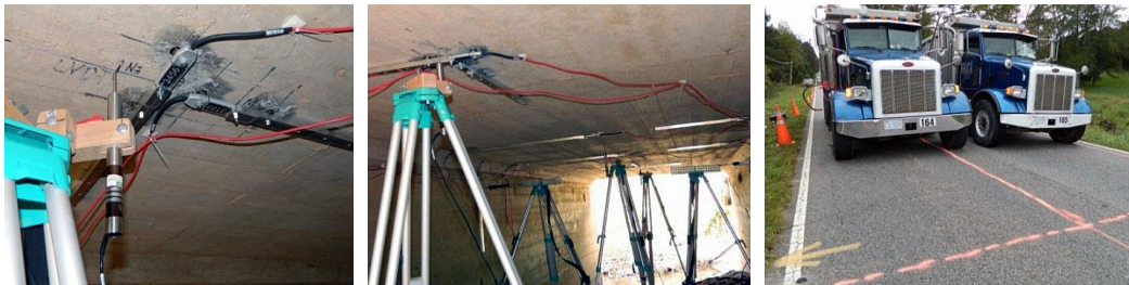
Field instrumentation and load testing of the reinforced concrete box culverts
