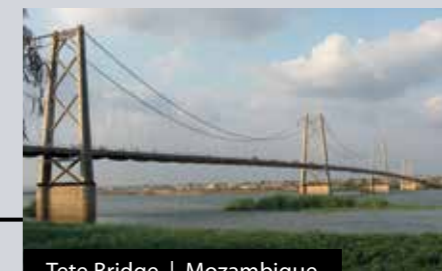
Tete Bridge | Mozambique
