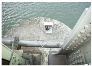
Figure 2: Sensor on the damaged pier
