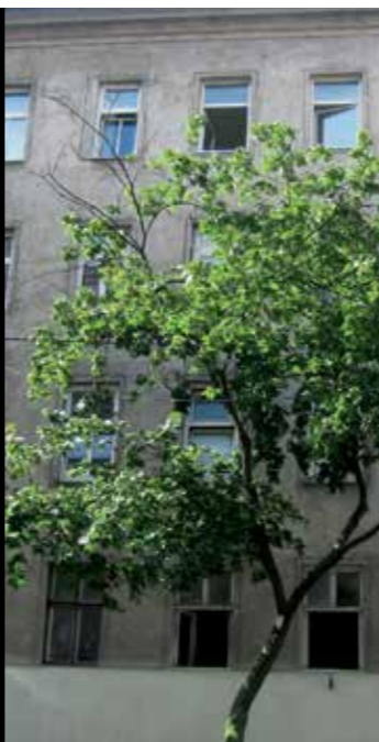
The building in Fendigasse (5 th district in Vienna) was excited by means of an unbalanced vibration exciter. The structural response was recorded at the facade by means of a Laser Doppler Vibrometer over four storeys. The figures (on the left) show different vibration responses at different frequencies.
